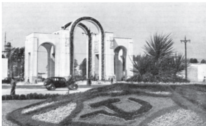
Figure 4. The new Main Entrance Arkhitektura SSSR, no. 9 (1939): 4.
