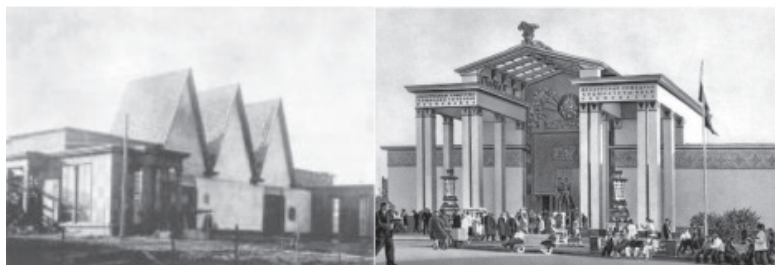
Figure 5. Belorussia Pavilion under construction (1937) and its new design (1939) Arkhitektura SSSR, no. 9 (1939): 23.
